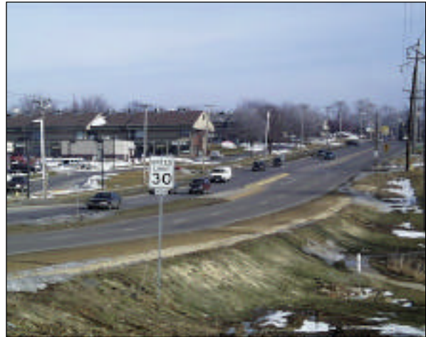
Section of managed access along the Douglas Avenue/Euclid Avenue corridor in Des Moines, Iowa. Result: very few left-turn-related crashes.
