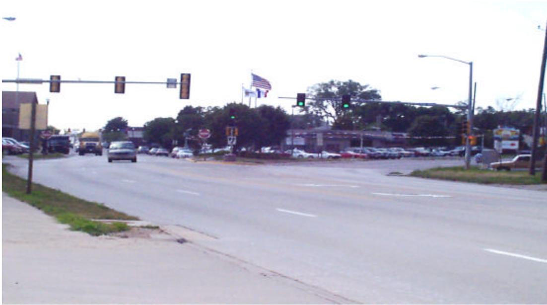
**Figure 2: State Street (US Highway 67) after the addition of a continuous two-way left-turn lane**
