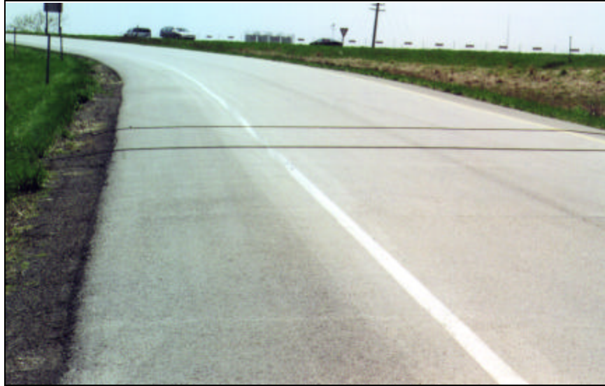
Figure 2.7. Pneumatic Road Tubes
