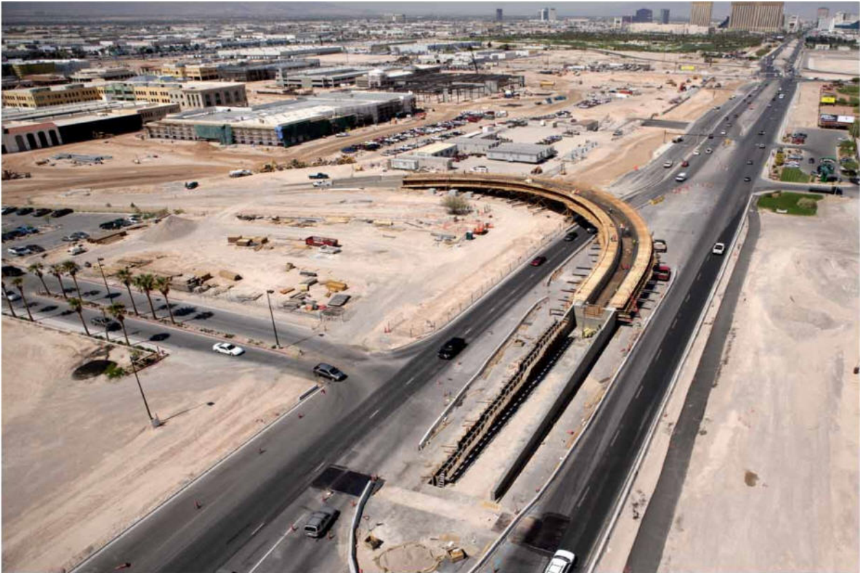
Figure 3. Aerial view of elevated left turn looking northbound on Las Vegas Boulevard
