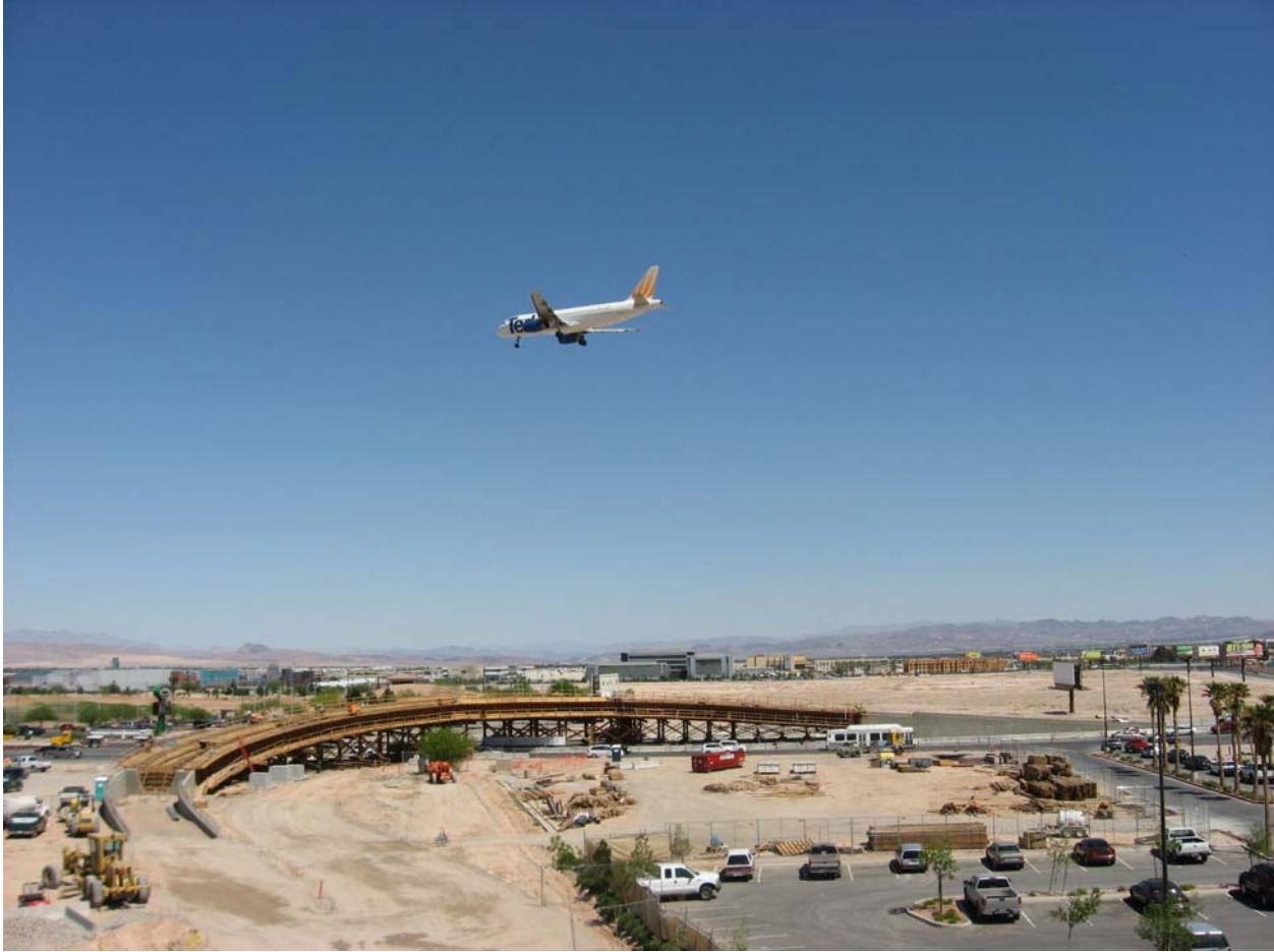
Figure 4. Looking east at the elevated left turn
