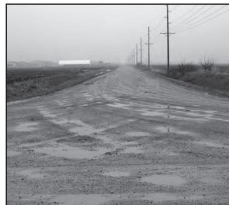
A muddy rural intersection with heavy traffic flow starts to show signs of spring damage.
