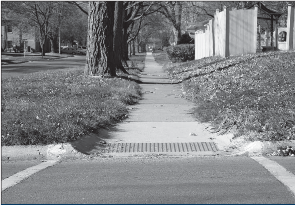
Complete street sidewalks should be four (and preferably five) feet wide, and should have curb ramps at crossings to be accessible to wheelchairs and strollers (photo courtesy of Bradley Grefe, CTRE at ISU).
