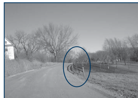
Circled above is the decorative fence that began Story County’s campaign to remove roadside safety hazards.
