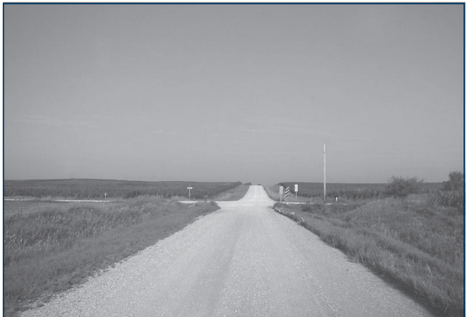
Ultra-low-volume unpaved rural intersections like this one may not need stop signs
